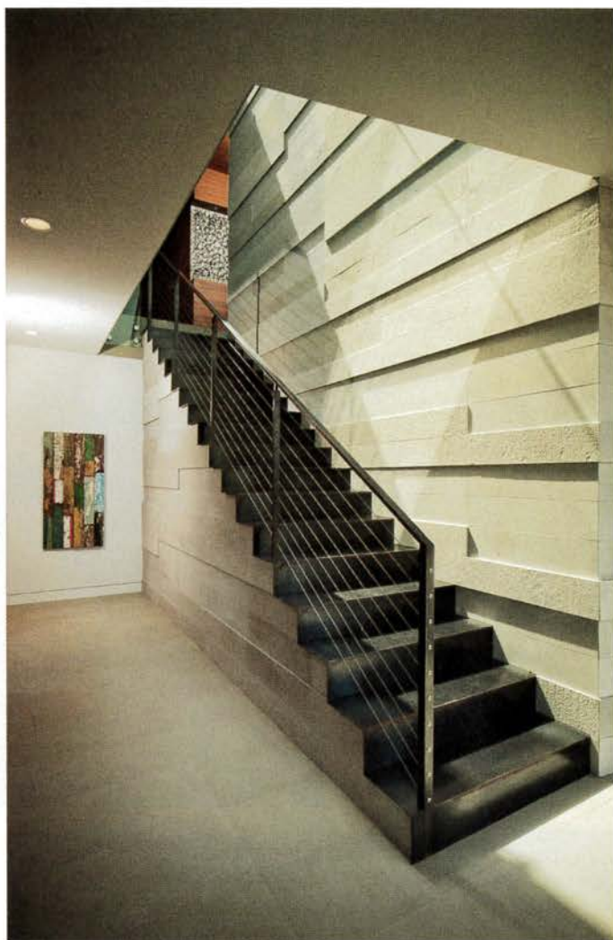
Staircase leading to the main level has rolled steel stairs and railing with a patina finish. The two-story wall is a composition of alternating bands of stone tile in three different textures lit by a large skylight above.
